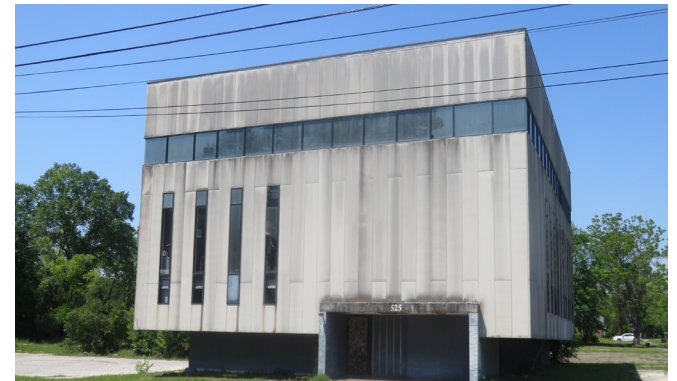
Blighted property along Augusta Ave.
