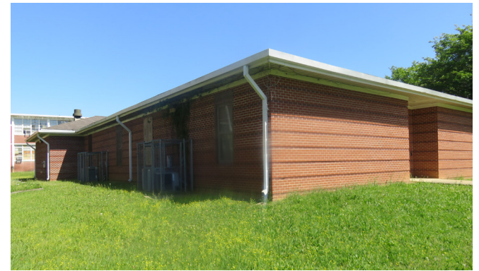
City of Montgomery Emergency Warming / Cooling Center
